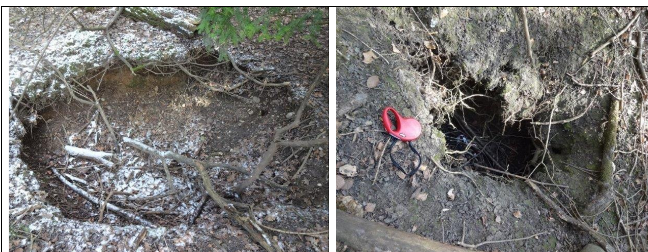
Plate 3: A fresh(ish) collapsed infill pit
